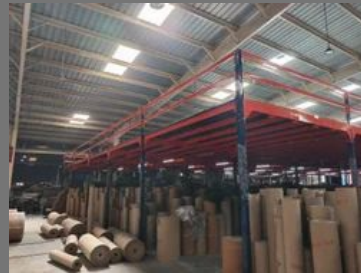
Mezzanine Floor Fabrication Service
