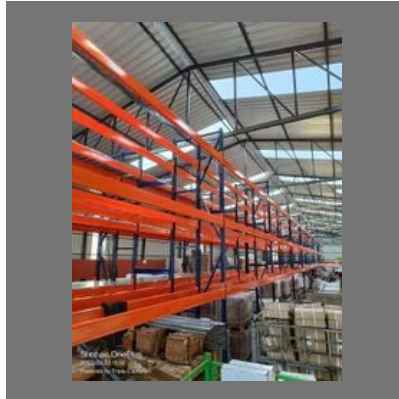
Warehouse Pallet Storage Racks
